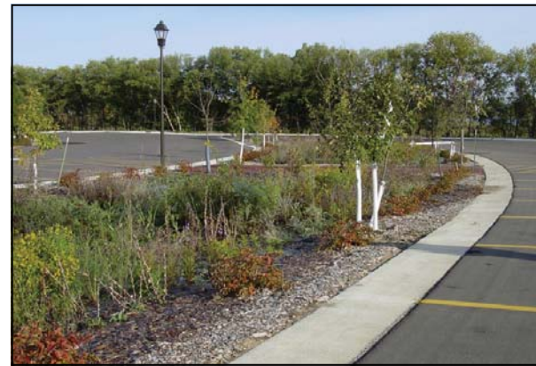
Bioretention cell utilized in a commercial parking lot
