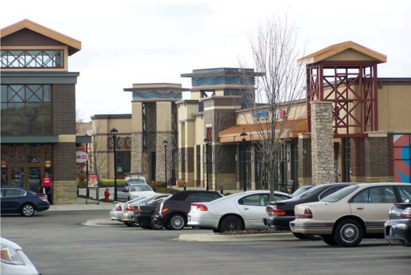
Bridgewater Falls Retail Development
