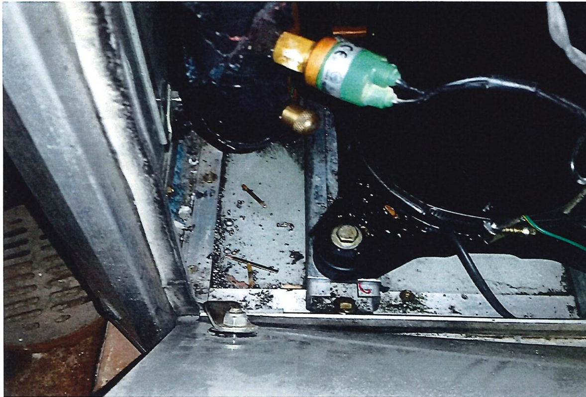
Parts left behind in unit
