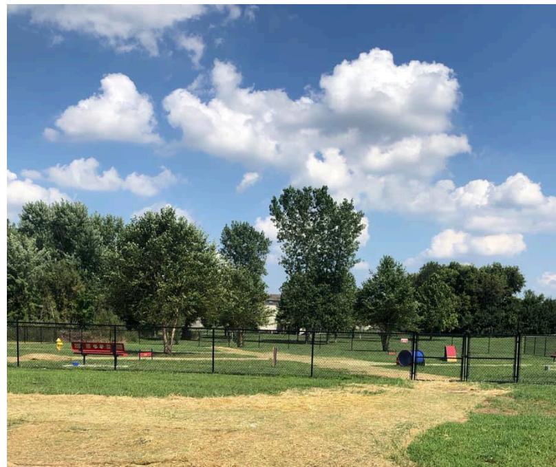
In-progress repairs and upgrades to Holly's Dog Park
